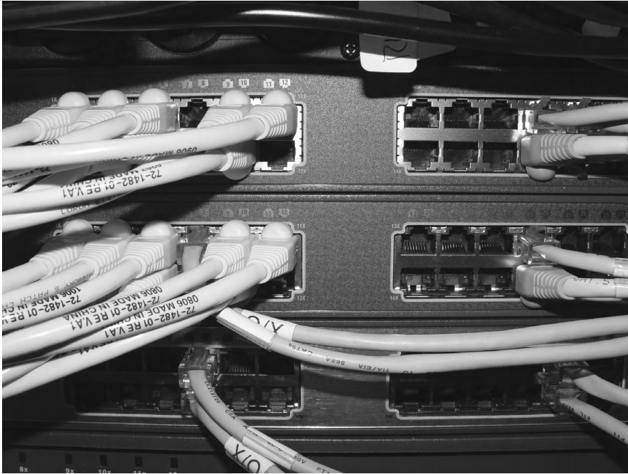
FIGURE 20.3 Rack-mounted switches
