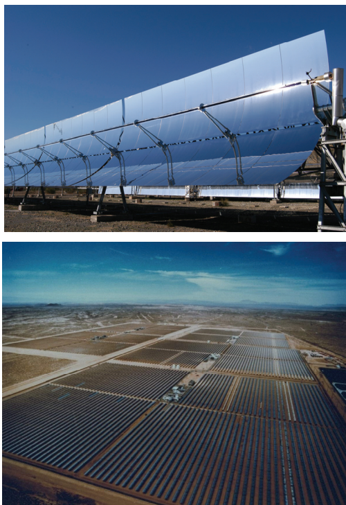
Figure 6. Parabolic trough solar collectors in Almería, Spain and California, USA (source: DLR and FVEE/PSA/DLR).
